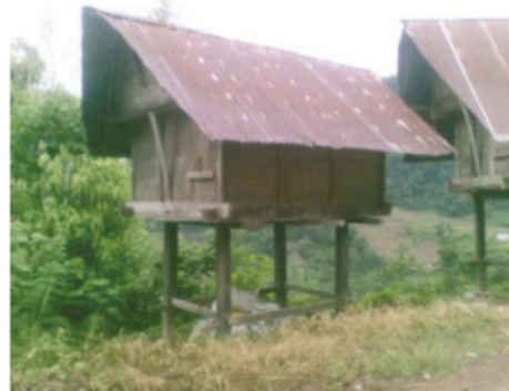
Fig. 3 — Granary (Landa) in Kendenan village, Enrekang district
